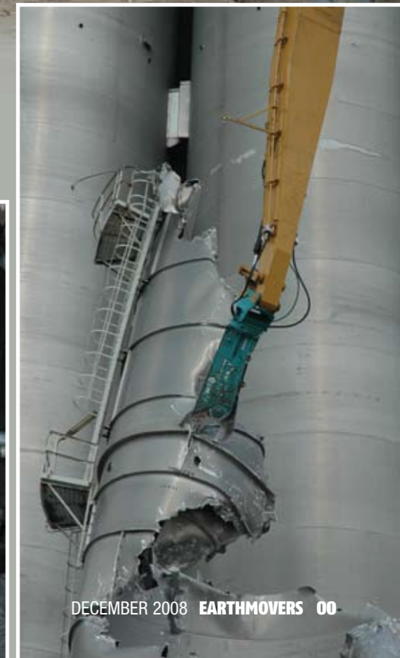
Right: Though currently fitted with a 3.5t tool, the rig is capable of carrying a five-tonne tool at full height and a 12t attachment to 80m.
