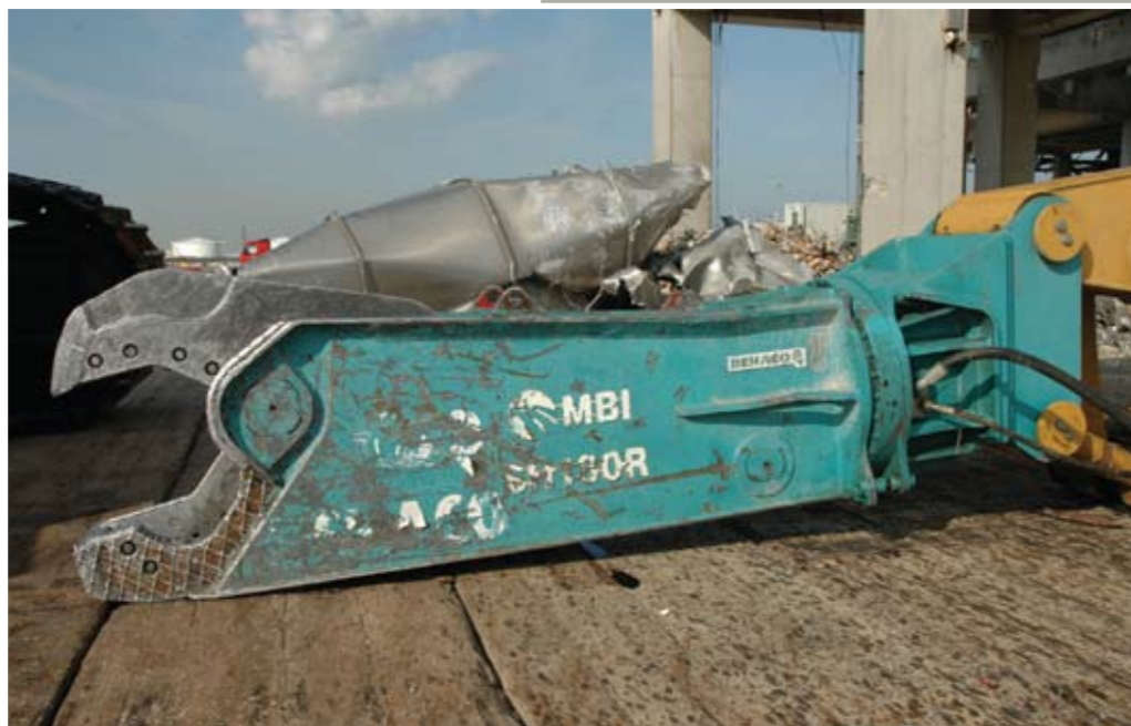
Below: The 90m rig is currently fitted with a 3.5-tonne Dehaco steel shear. Here it munches through the aluminium, which varies in thickness from 1cm to 4cm.
